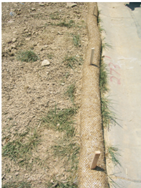
Drive stakes every 3-4 feet along the filter log. Photo credit: Barry Tanning, Tetra Tech.
