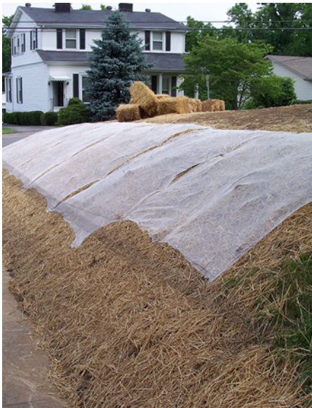
Slope stabilization using mulch and mulch nets. Photo credit: Barry Tanning, Tetra Tech
