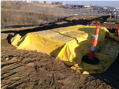
Cover materials using tarps or plastic sheeting to prevent precipitation from contacting construction site materials. Direct work crews to replace material stockpile covers at the end of the day and before rain. Photo credit: Barry Tanning, Tetra Tech
