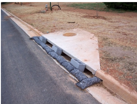
Typical rock bag inlet protection installation. Photo credit: Barry Tinning, Tetra Tech
