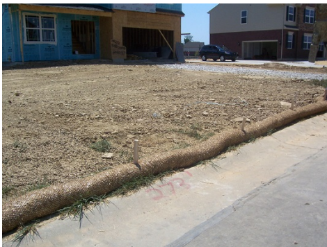
Make sure filter log stakes are spaced to prevent undercutting or bypasses. Leave stake tops extended along sections to prevent drive-overs. Photo credit: Barry Tanning, Tetra Tech
