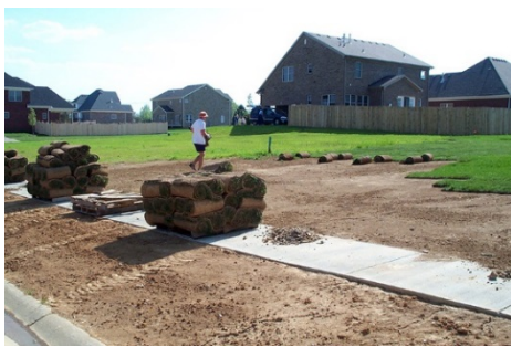
Photo of sod being installed at a residential site. Photo credit: Barry Tanning, Tetra Tech
