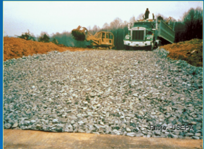
Good Gravel Over Geotextile
