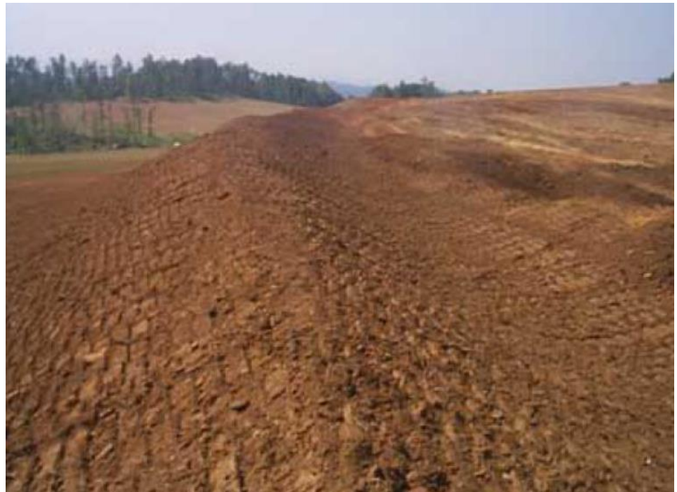
Diversion near the top of a slope
