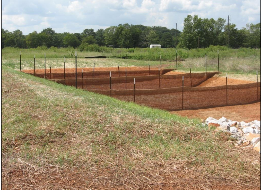
Example of porous baffle made of 700 g/m 2 coir erosion blanket as viewed from the inlet
